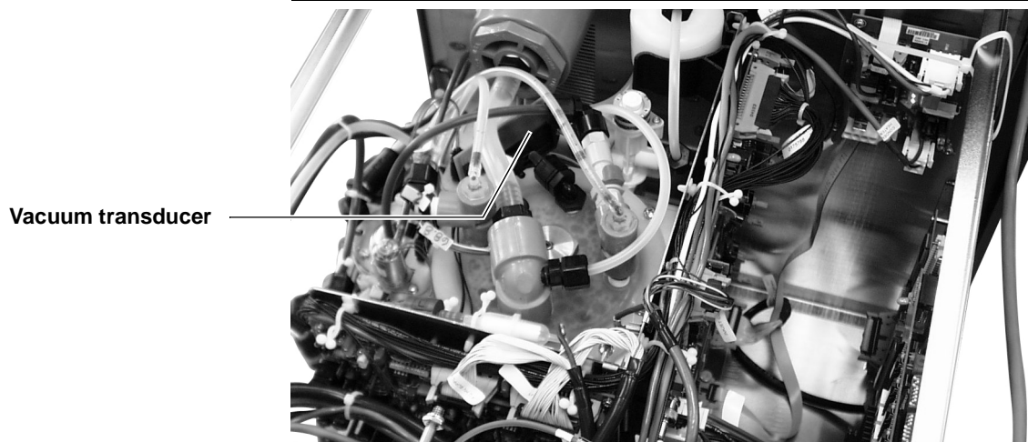
Figure 5.143 Vacuum transducer location, 5122
