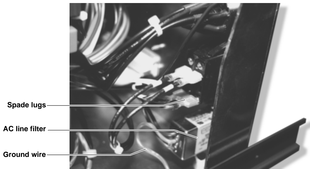
Figure 5.17 AC line filter removal
