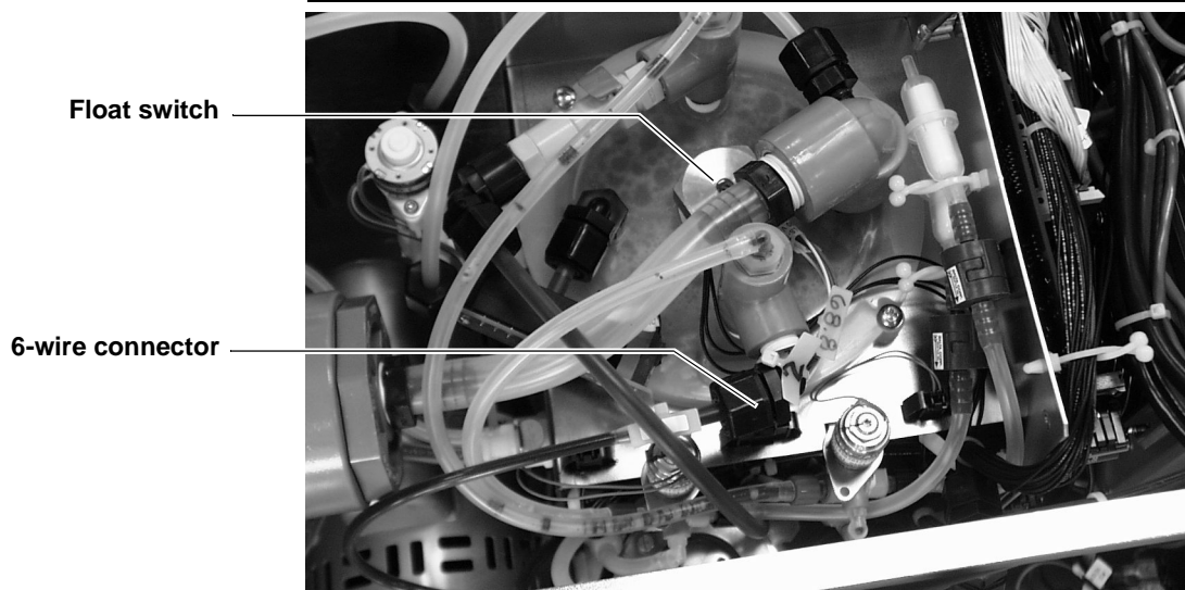
Figure 5.104 Float switch location, 5122
